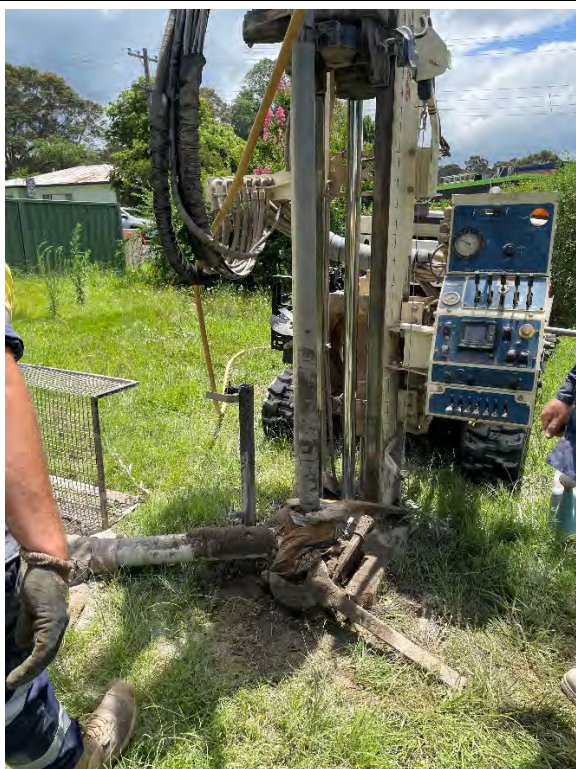
Figure 1. Drilling of BH04, evidence of moisture on rod visible.
