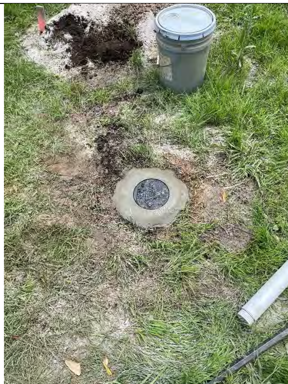
Figure 2. Installation of BH04, gatic cover fixed I place.
